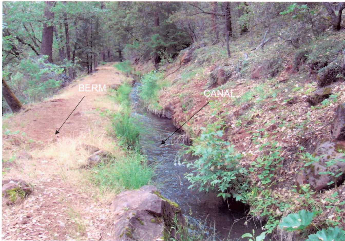
Mill Creek Canal - Earthen Section
