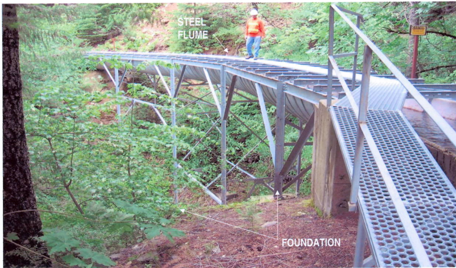
Kilarc Main Canal – Steel Flume
