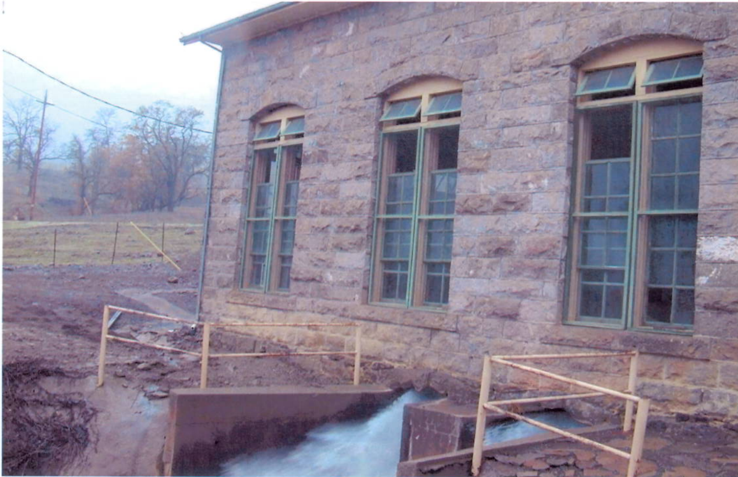
Cow Creek Powerhouse
