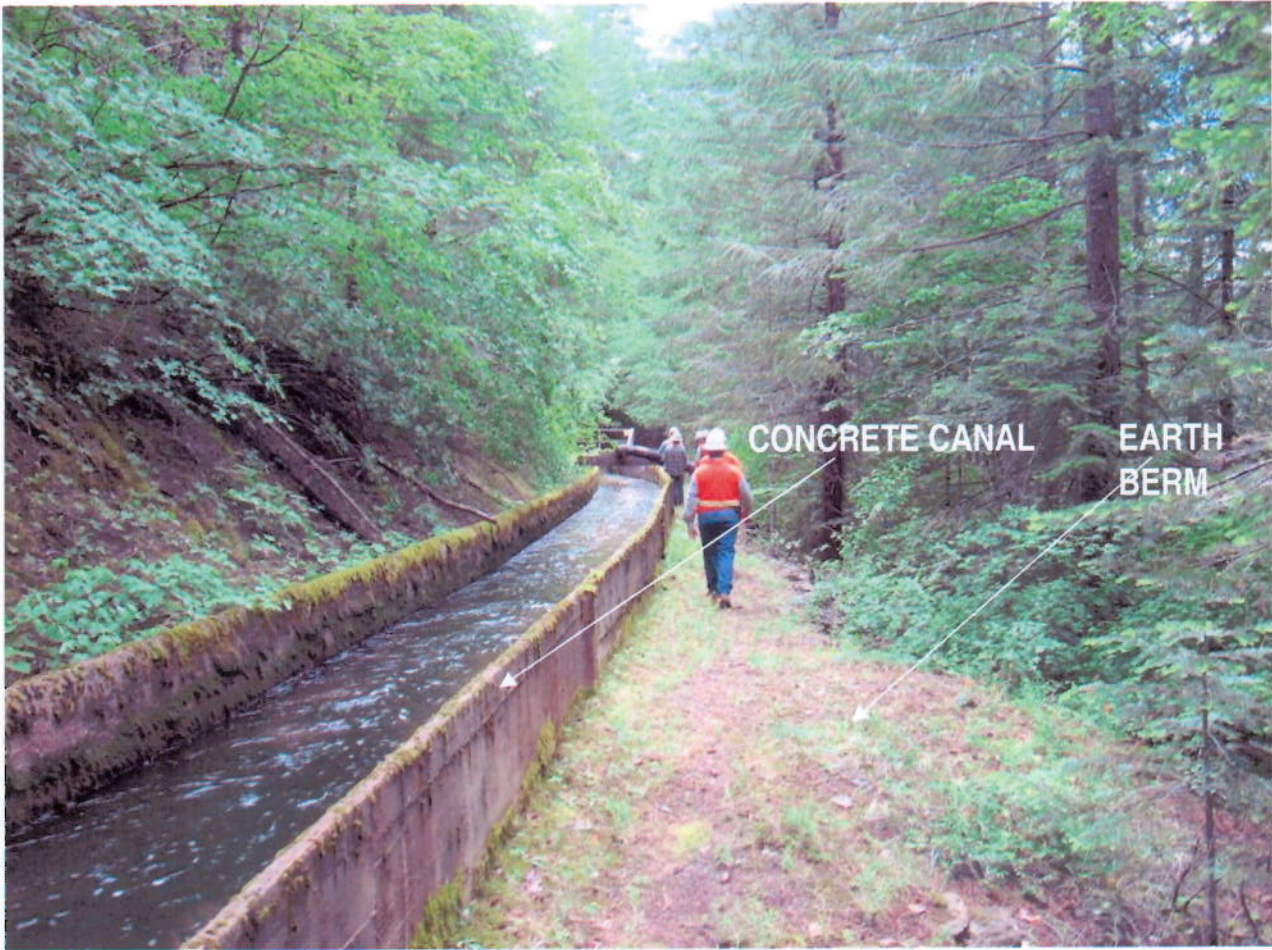
Kilarc Main Canal – Concrete Section
