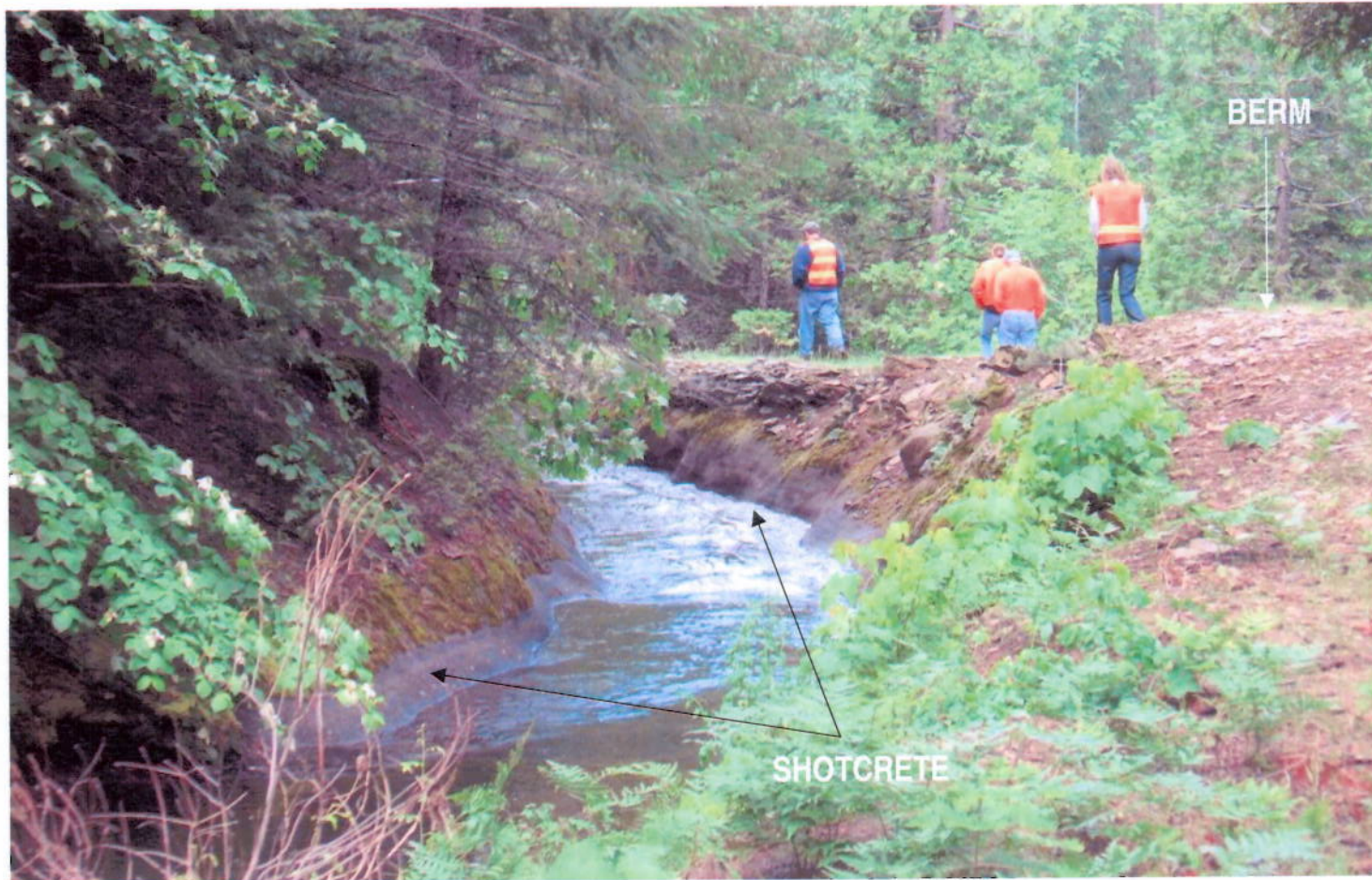
Kilarc Main Canal – Shotcrete Lined Section
