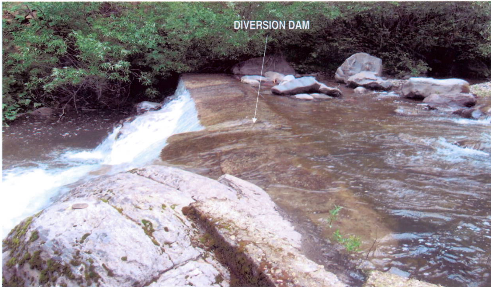
Kilarc Diversion Dam
