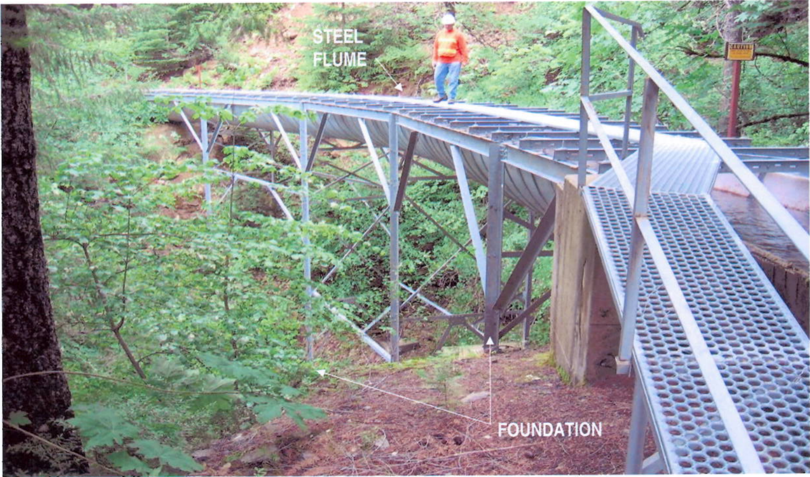
Kilarc Main Canal – Steel Flume
