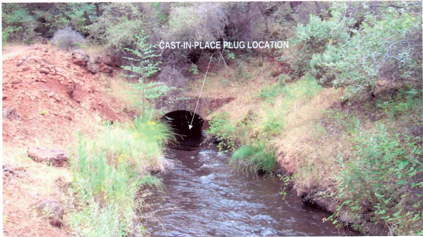
South Cow Creek Canal - Tunnel
