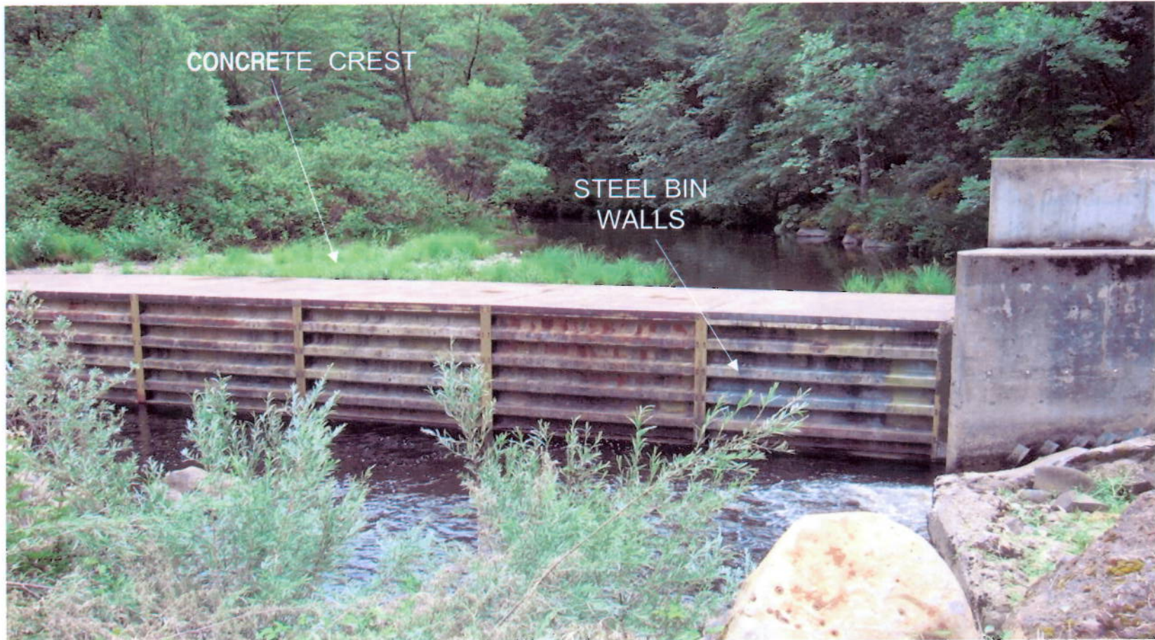
South Cow Creek Diversion Dam
