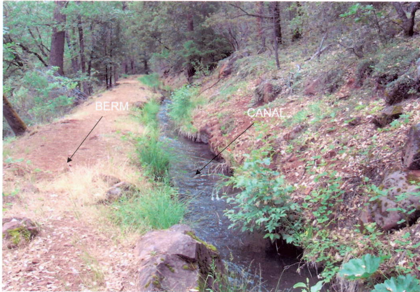
Mill Creek Canal - Earthen Section
