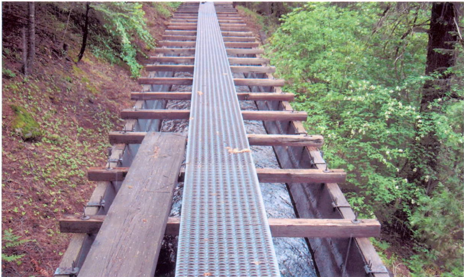
Kilarc Main Canal – Wooden Flume
