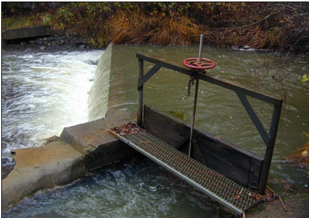
Photograph E.2.3-2. Mill Creek Diversion and Dam
