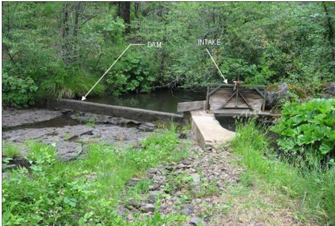
Photograph 2.3.1-1 Mill Creek Diversion – Dam and Canal Intake
