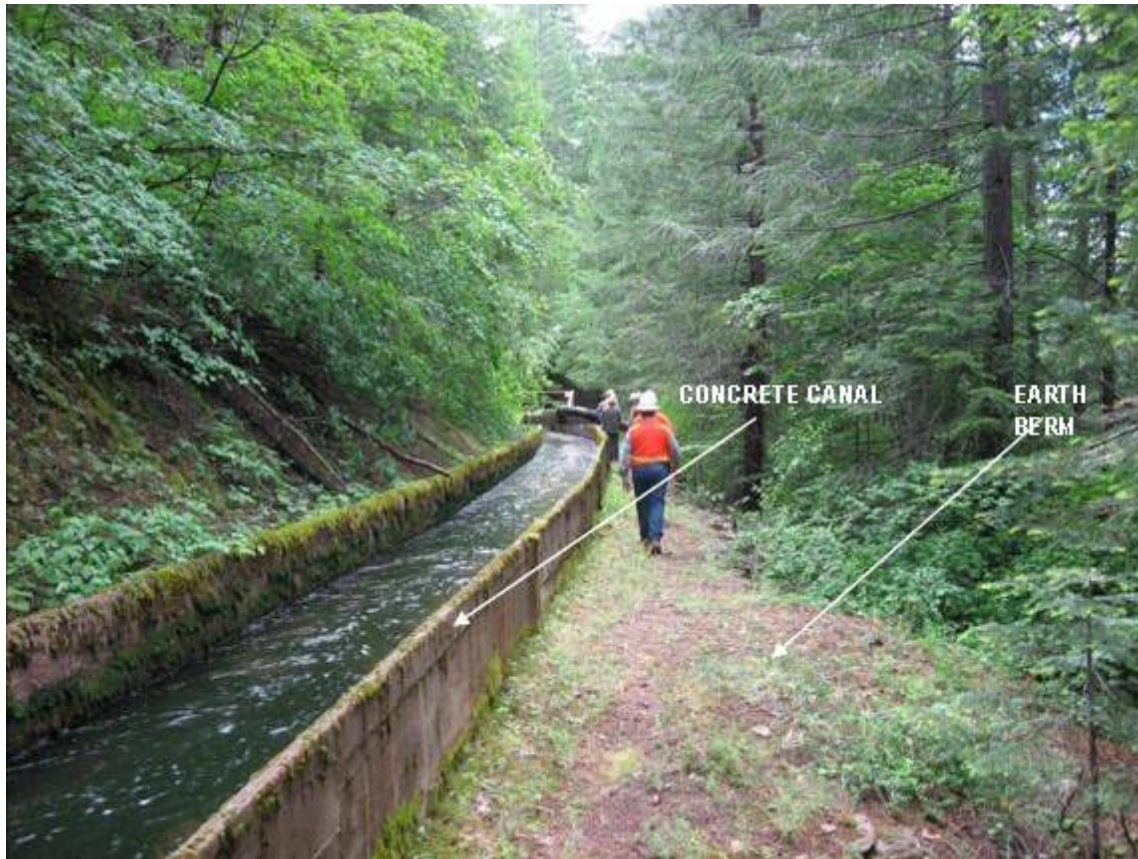
Photograph 2.2.4-1a Kilarc Main Canal – Concrete Section
