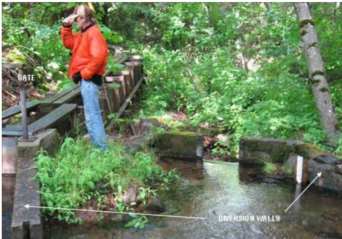
Photograph 2.2.2-1a South Canyon Creek – Diversion and Canal Inlet
