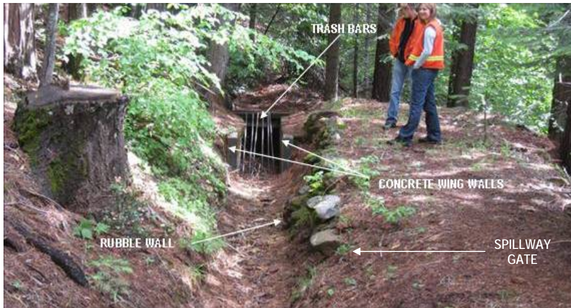
Photograph 2.2.2-1d South Canyon Creek – Canal Siphon Inlet
