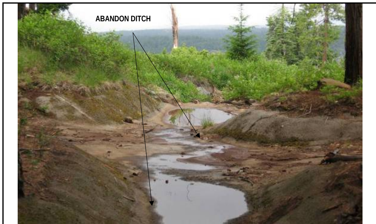
Photograph A-10. Kilarc Forebay Spill Channel.
