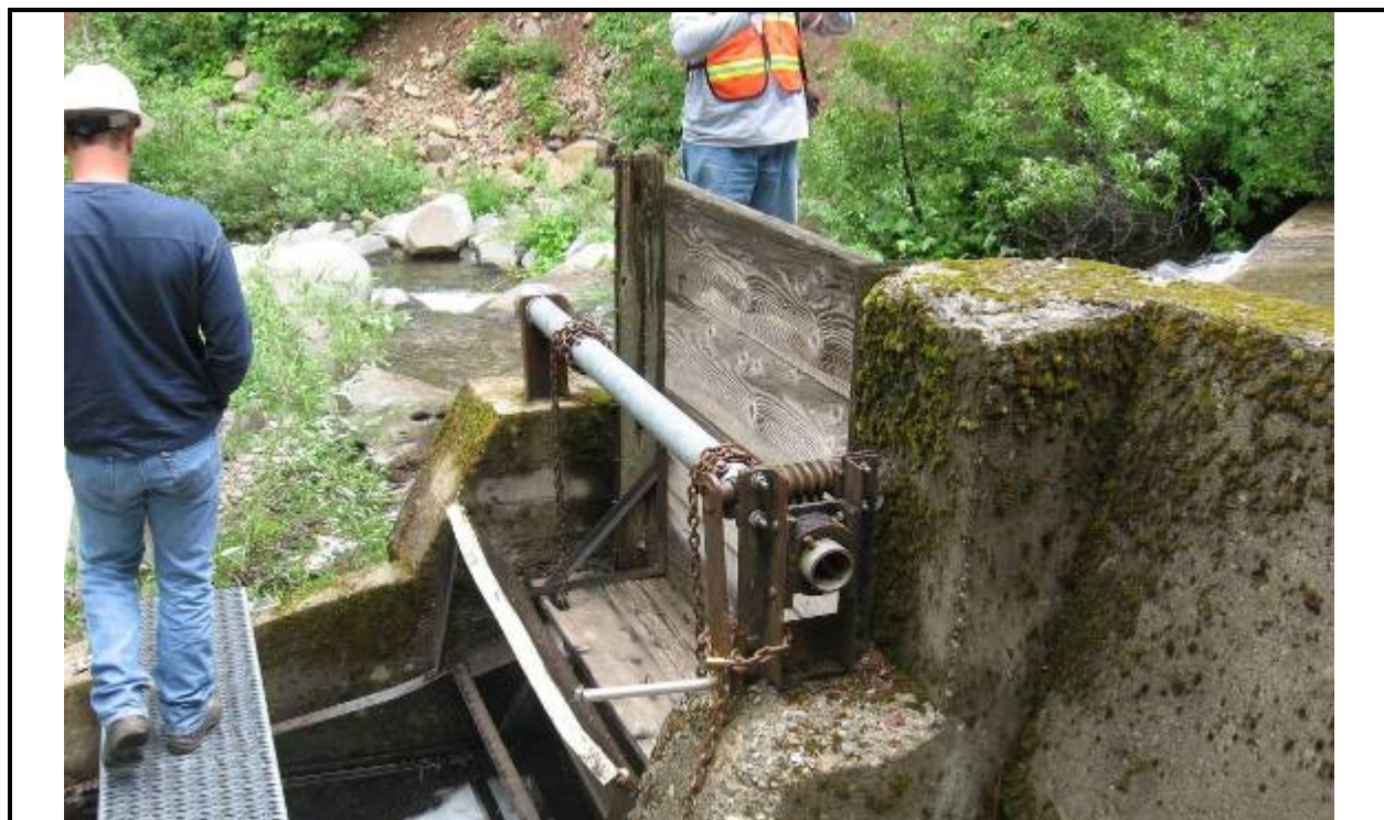
Photograph A-2. Kilarc Main Canal Intake.
