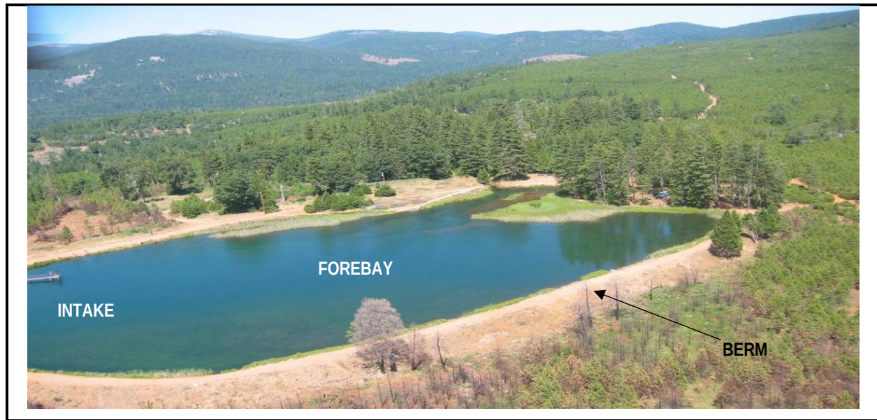
Photograph A-9. Kilarc Forebay Spill Channel.
