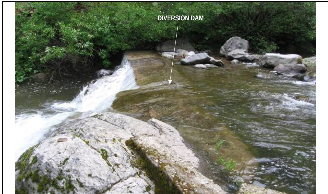
Photograph A-3. Kilarc Main Canal Diversion.
