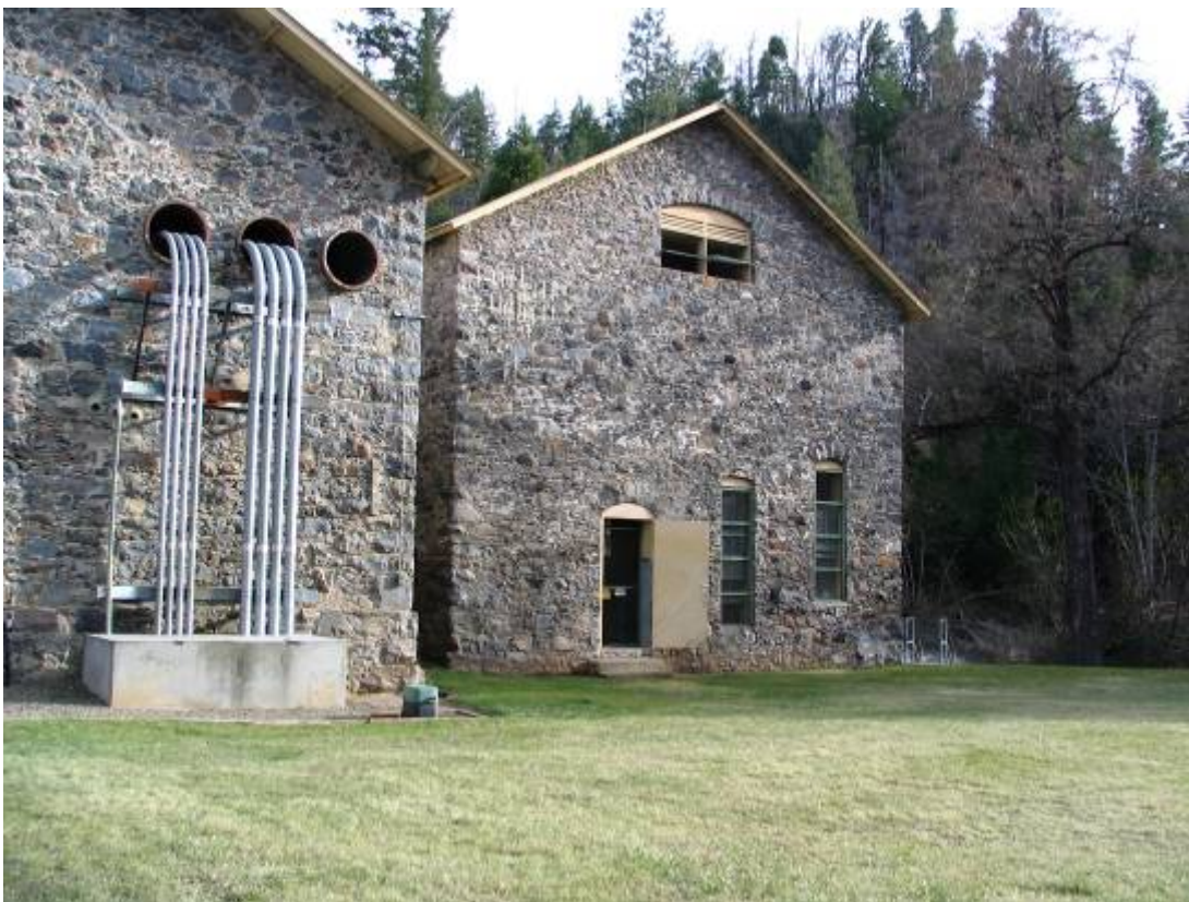
Photograph 1.1-1a Kilarc Powerhouse and Adjacent Land
