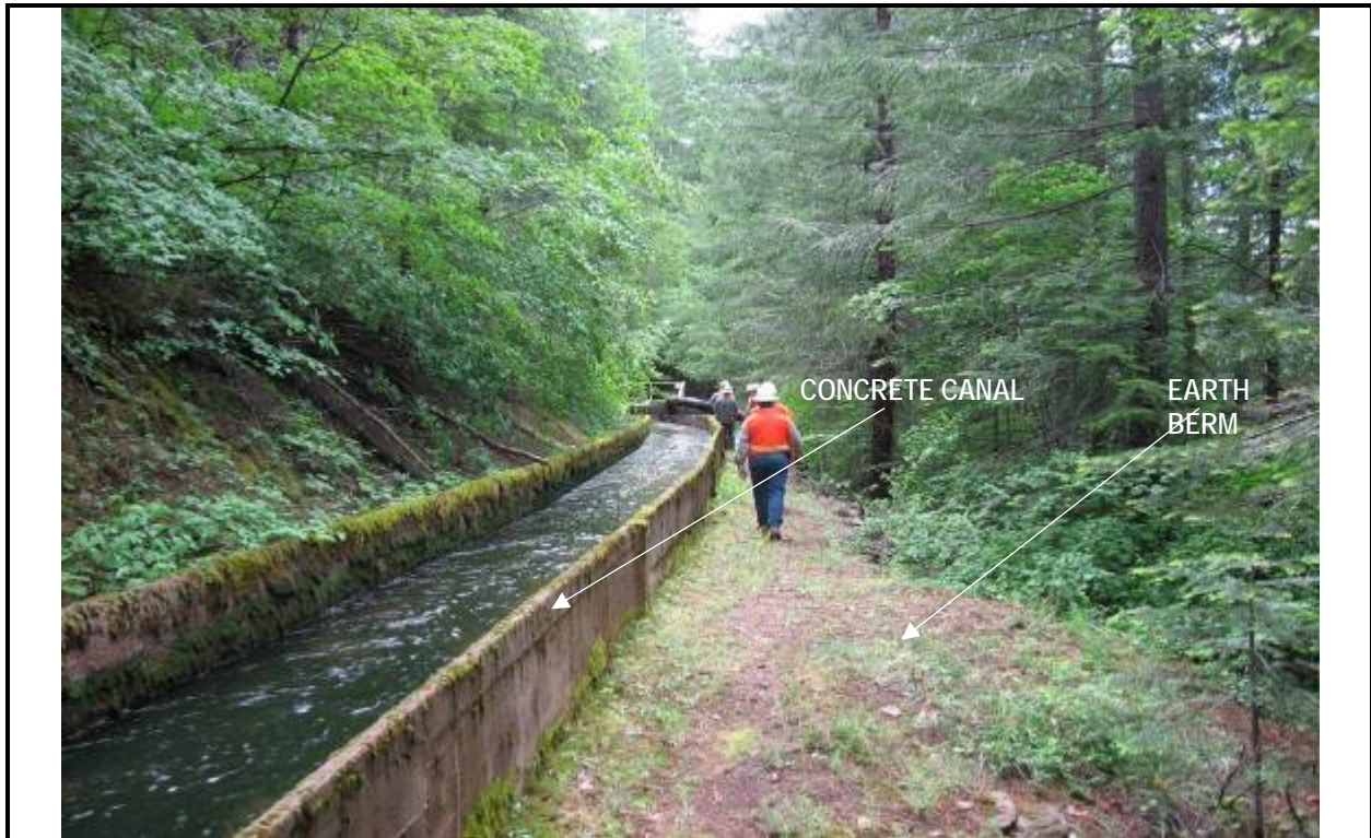
Photograph A-5. Concrete Lined Section of Kilarc Main Canal.
