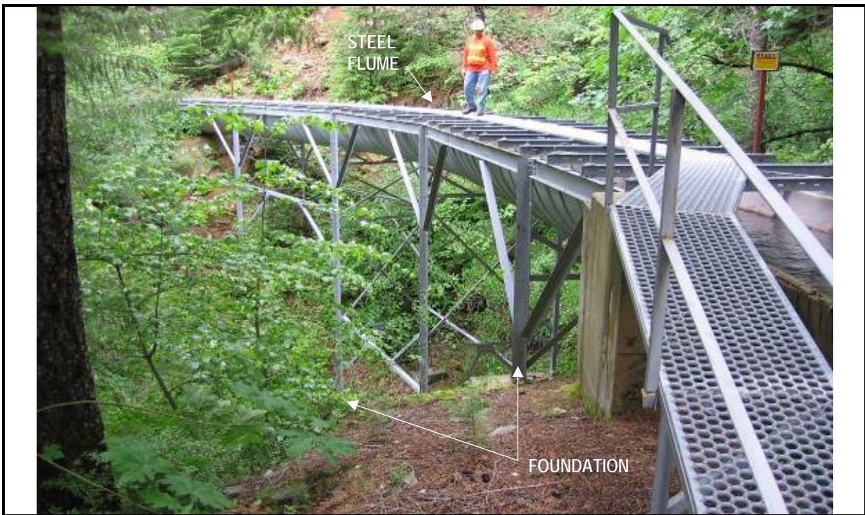
Photograph A-8. Steel Flume of Kilarc Main Canal.
