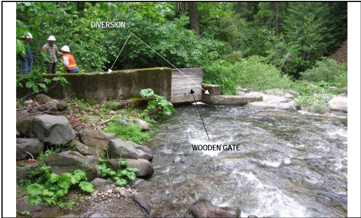
Photograph A-1. Kilarc Main Canal Diversion from Upstream.
