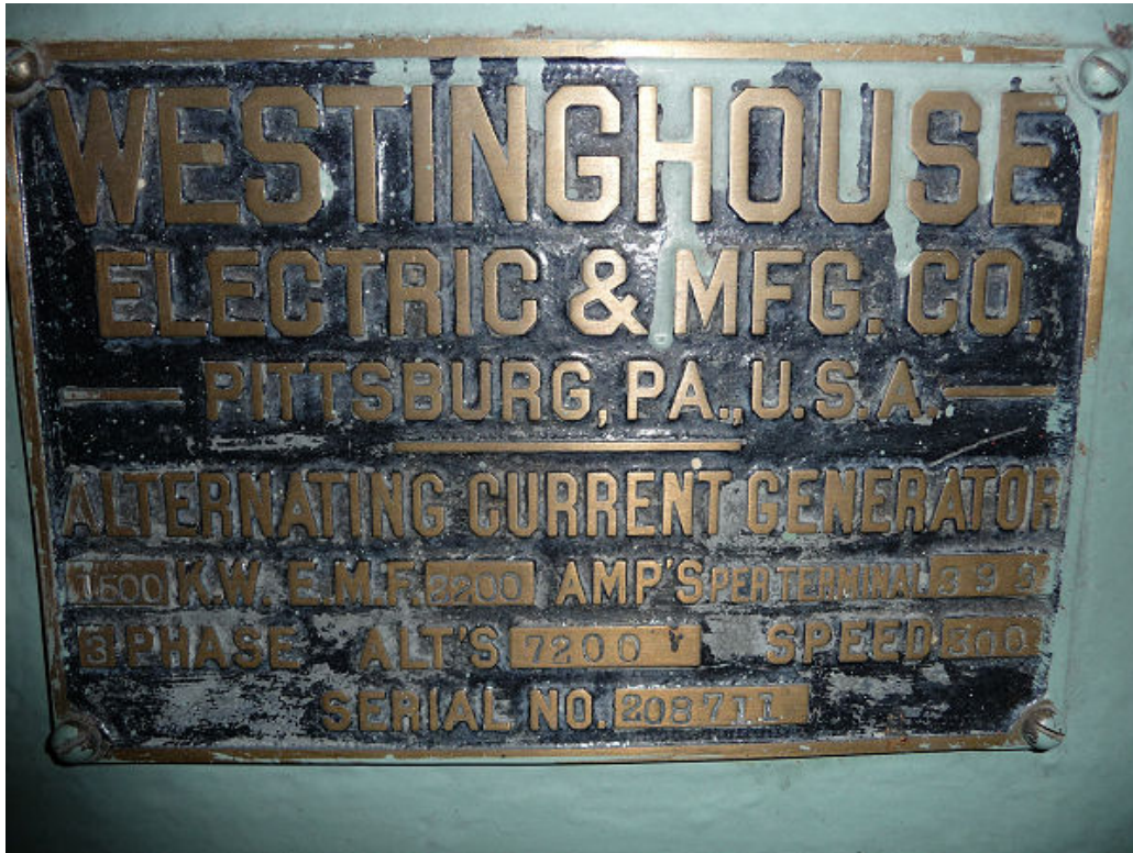
Picture 1 – Kilarc Powerhouse Plate
